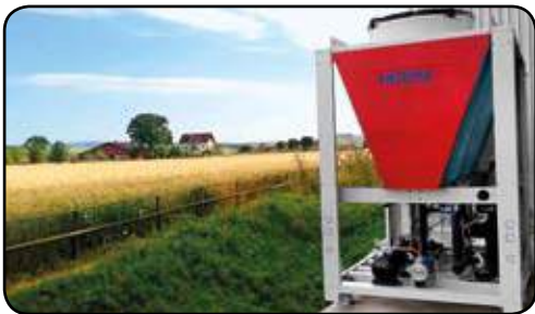
* Modular reversible air to water heat pump installed in Switzerland for space heating/cooling. 105kW @ +45°C LWT
